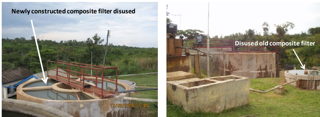
Plate 4: Filter Composite units
