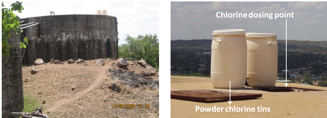
Plate 17: Bomani Reservoir and chlorine dosing point
