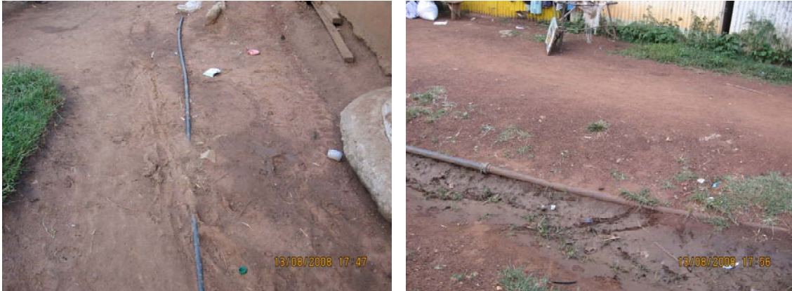
Plate 11: Pipes laid on the surface in Bondo town
