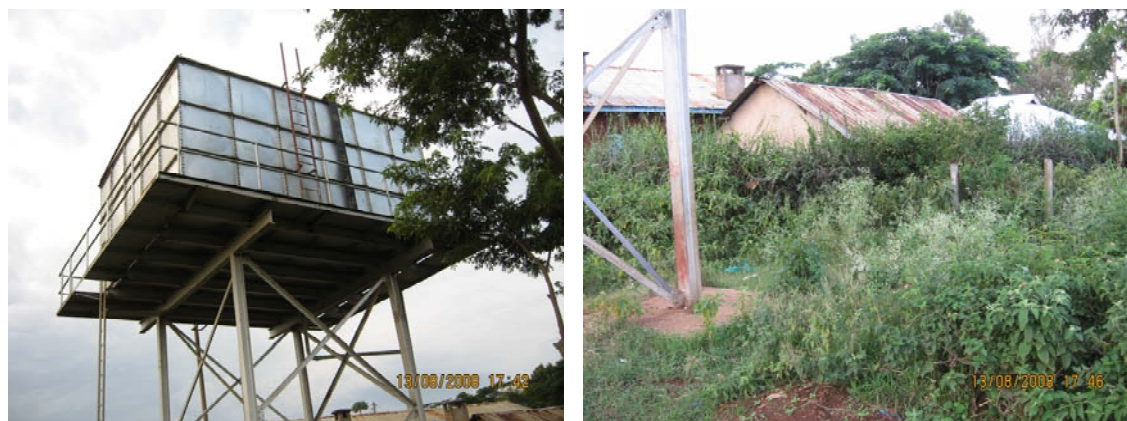
Plate 8: Elevated reservoir for Bondo Water Supply area
